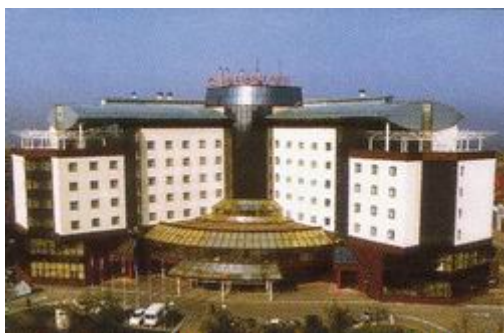
Hotel complex in Samara “Renaissance Samara Hotel Leasing” LLC Novo-Sadovaya Street 162v
